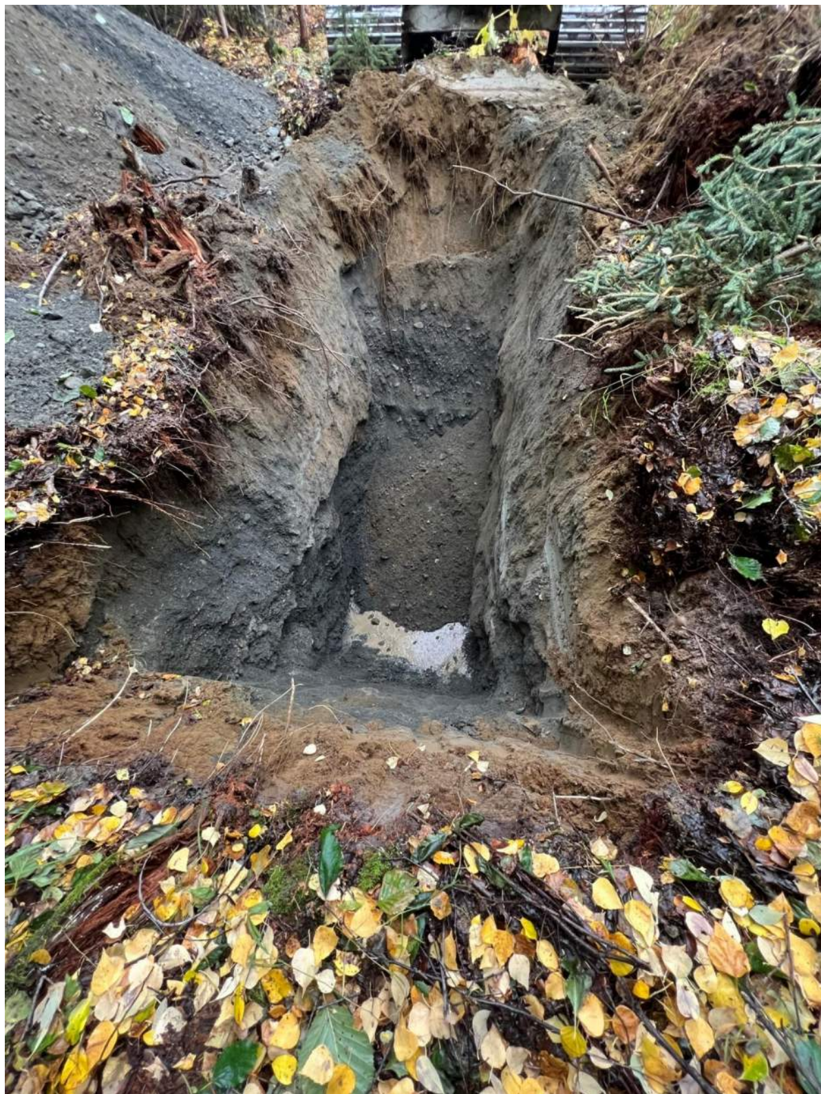
Photo A - 15: Test Pit TP15
