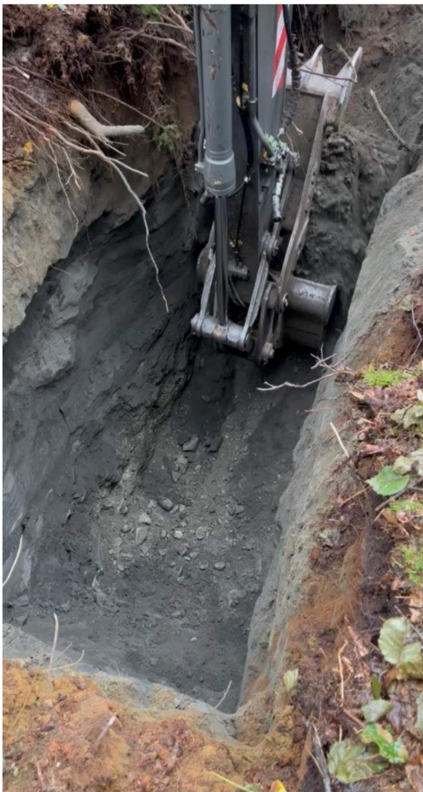
Photo A - 21: Test Pit TP21
