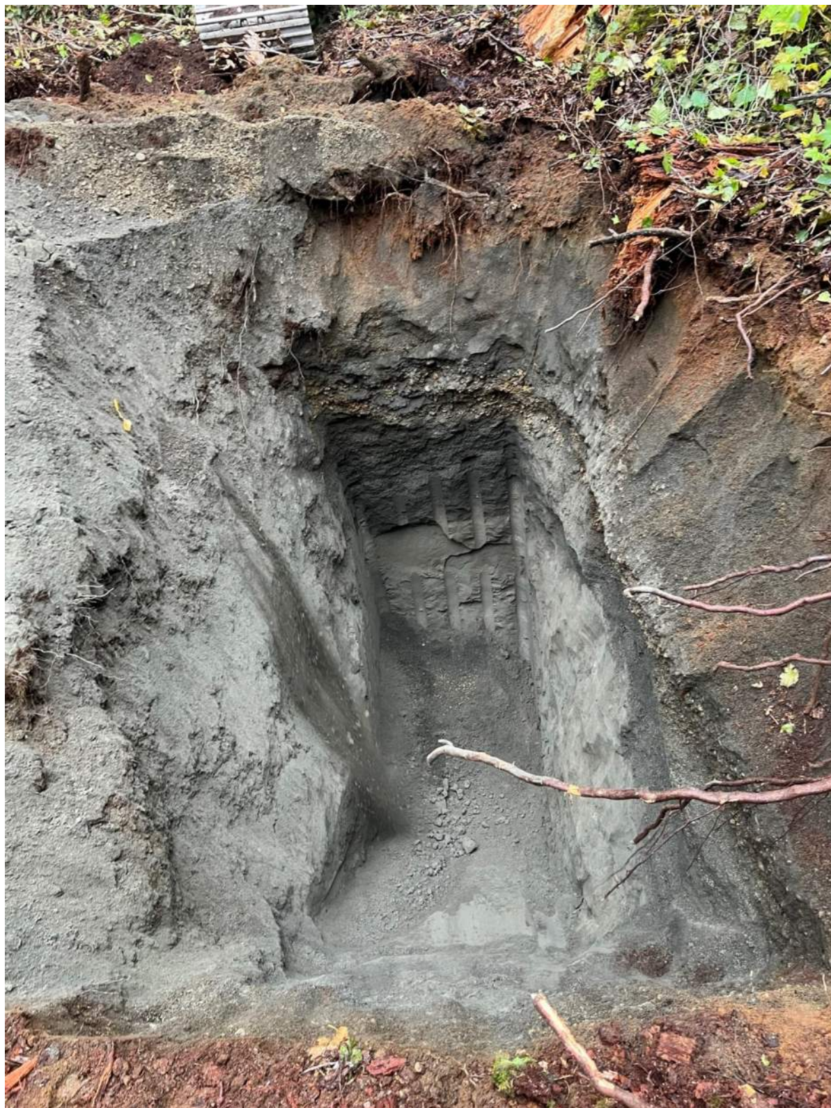
Photo A - 20: Test Pit TP20
