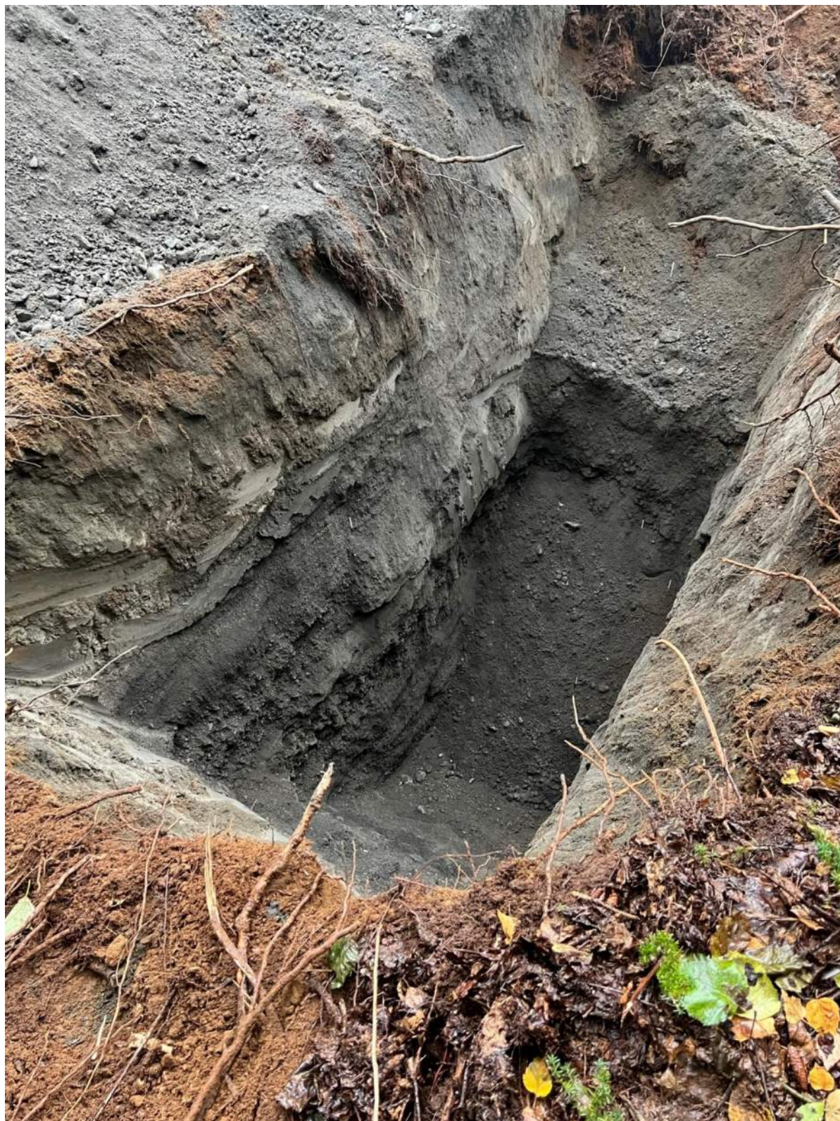
Photo A - 23: Test Pit TP23
