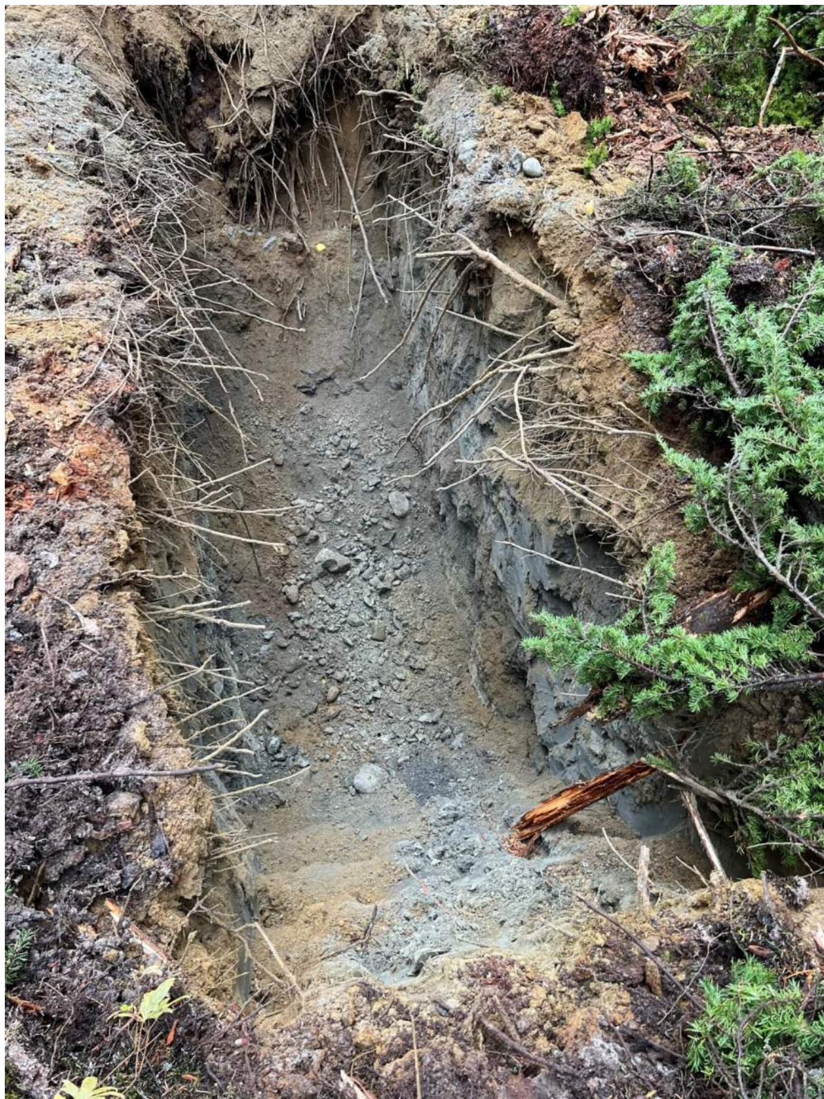
Photo A - 39: Test Pit TP39
