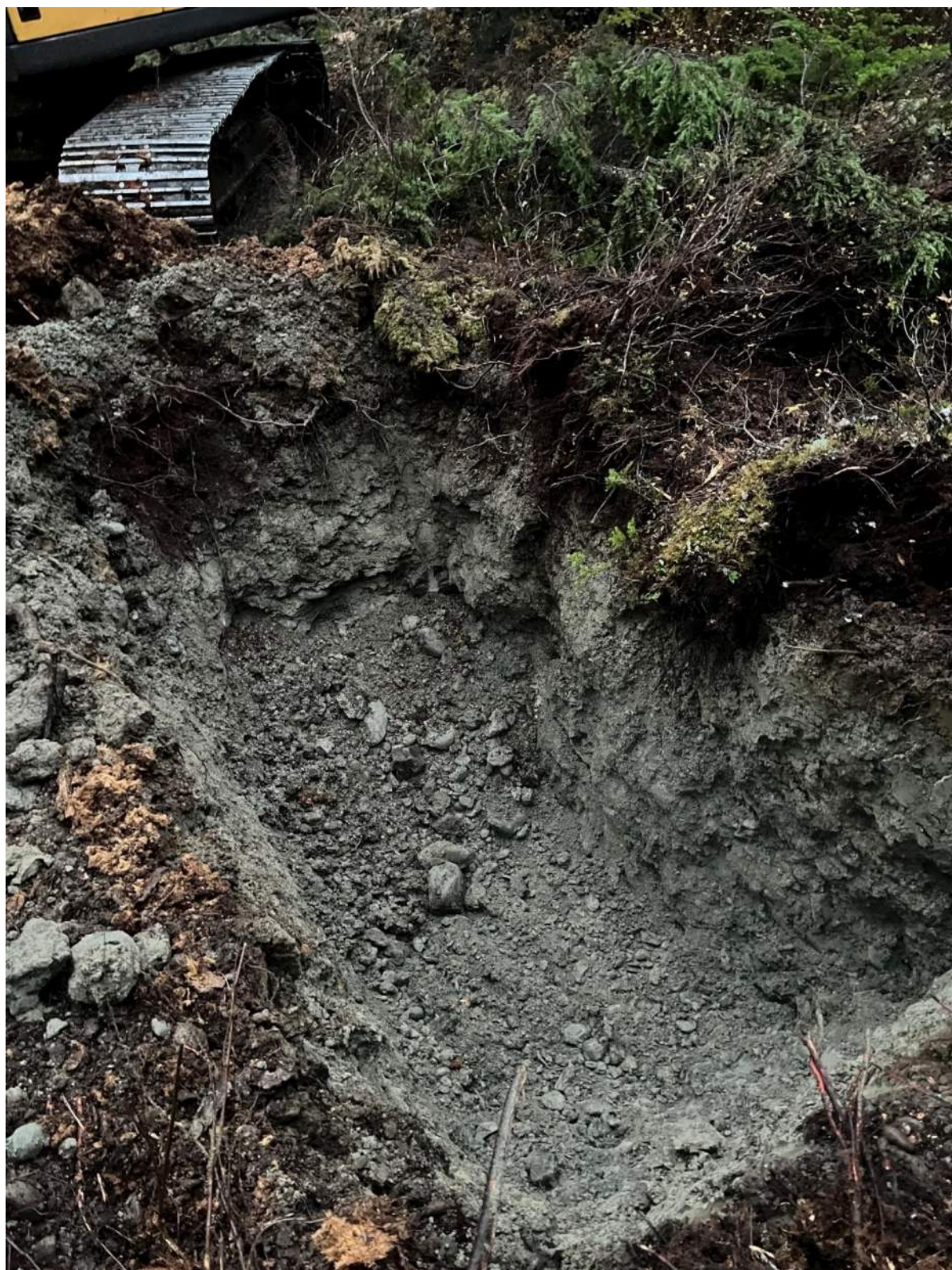
Photo A - 33: Test Pit TP33
