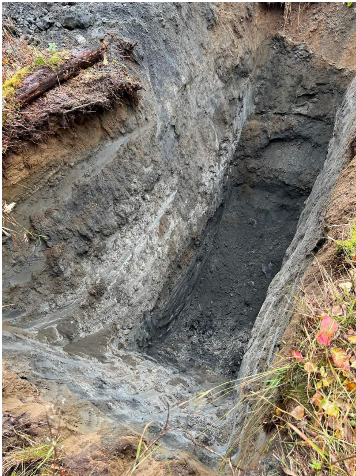
Photo A - 13: Test Pit TP13
