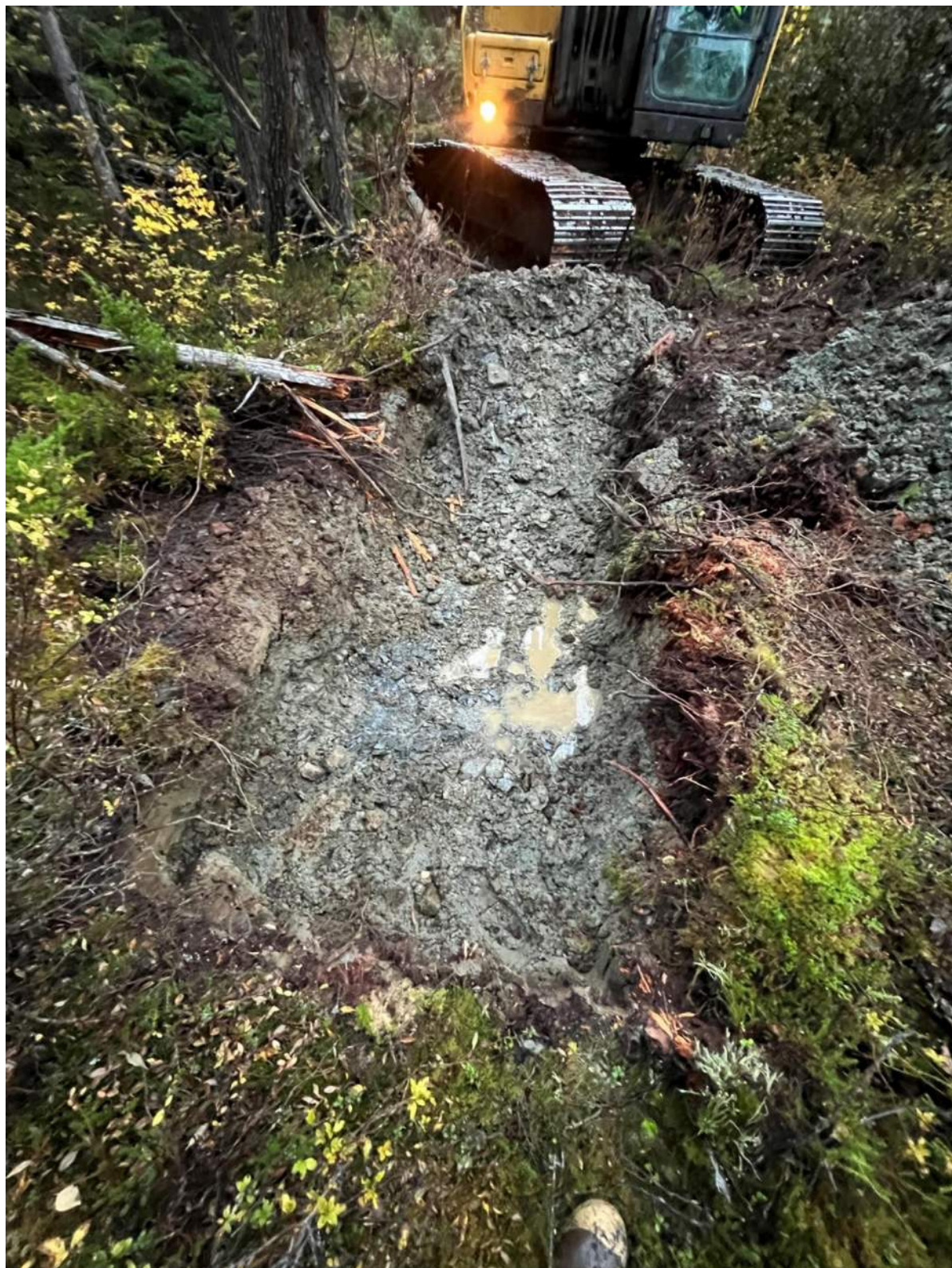
Photo A - 35: Test Pit TP35
