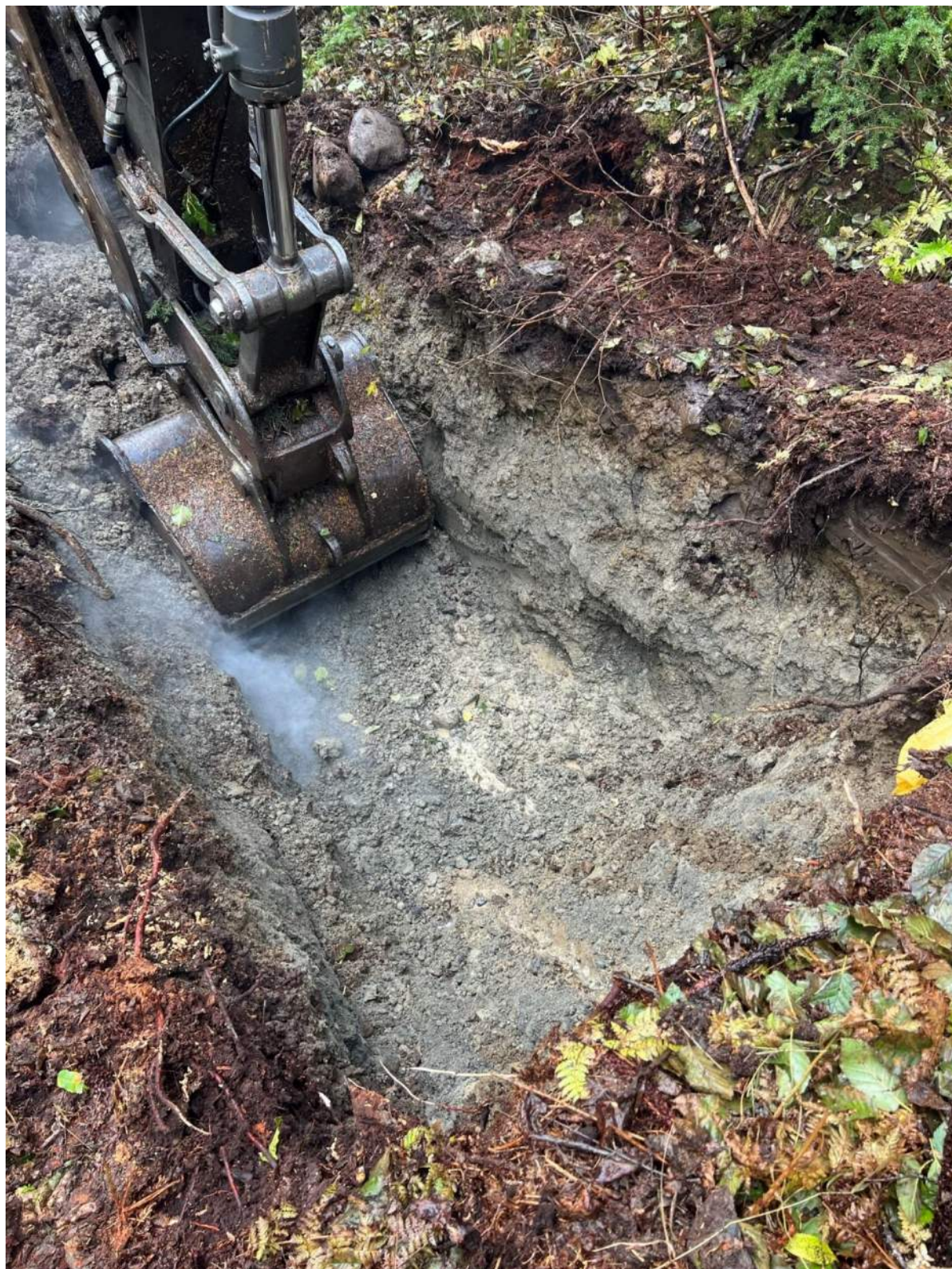
Photo A - 29: Test Pit TP29
