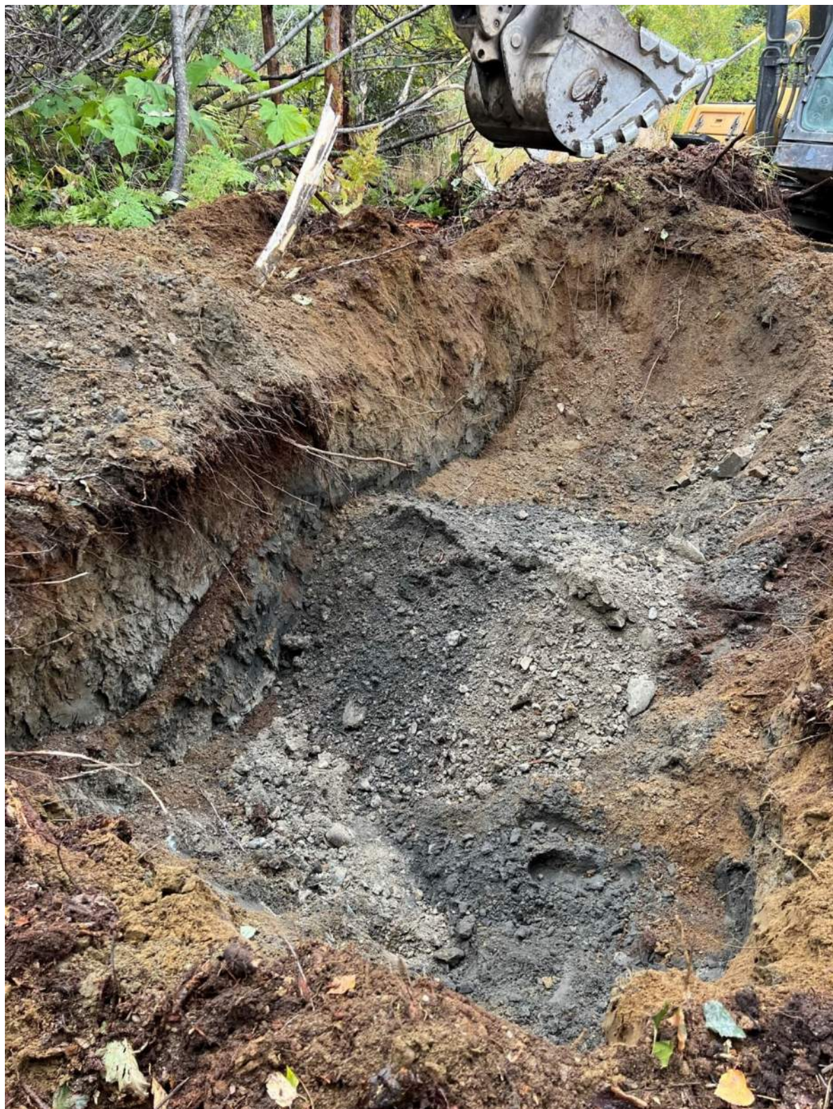
Photo A - 7: Test Pit TP7
