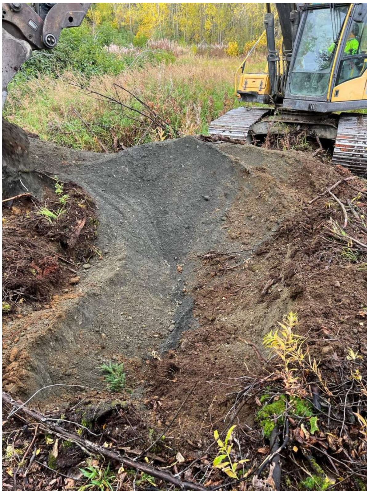
Photo A - 18: Test Pit TP18 In Progress
