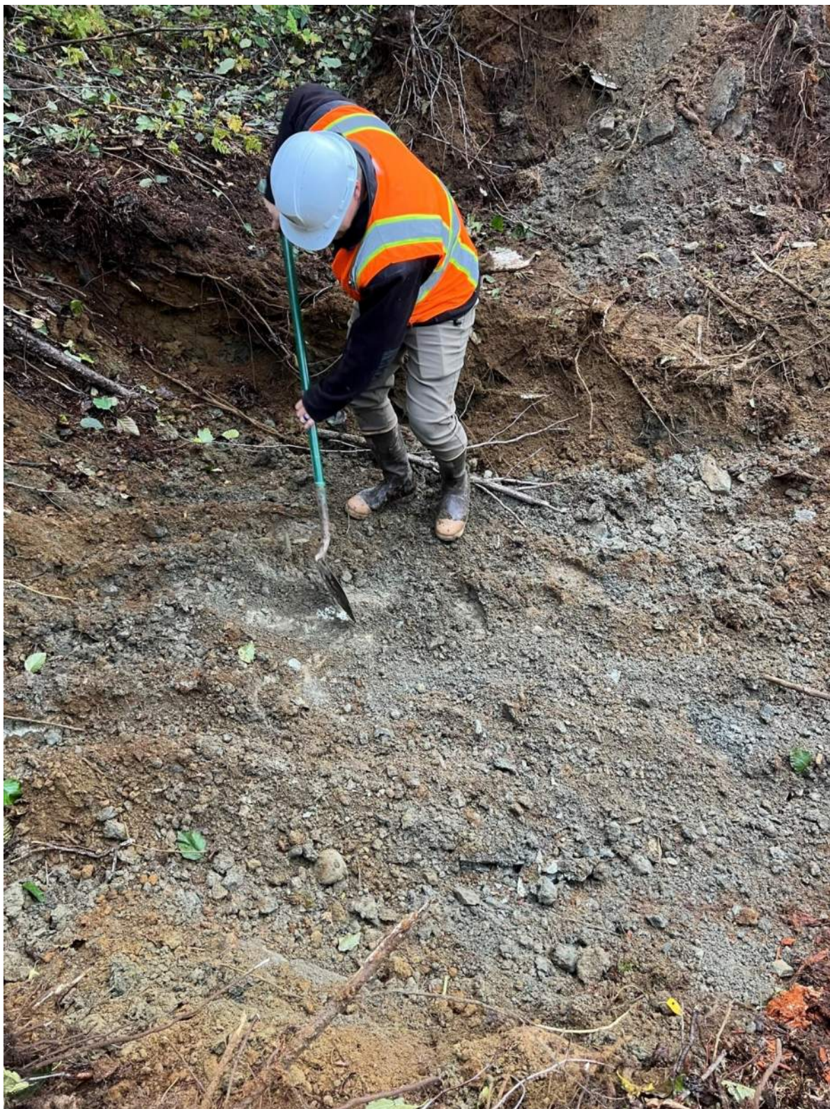
Photo A - 6: Test Pit TP6
