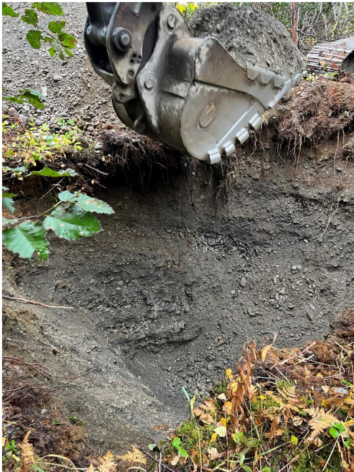
Photo A - 2: Test Pit TP2
