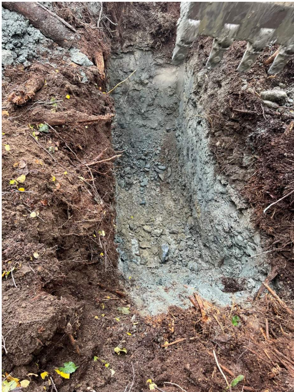
Photo A - 11: Test Pit TP11
