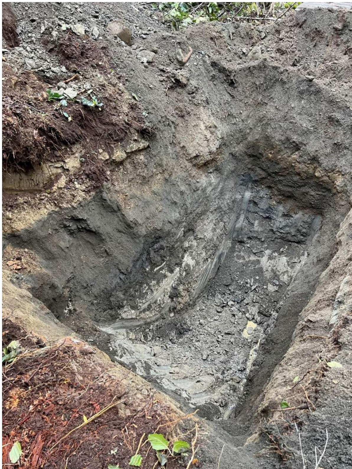
Photo A - 5: Test Pit TP5
