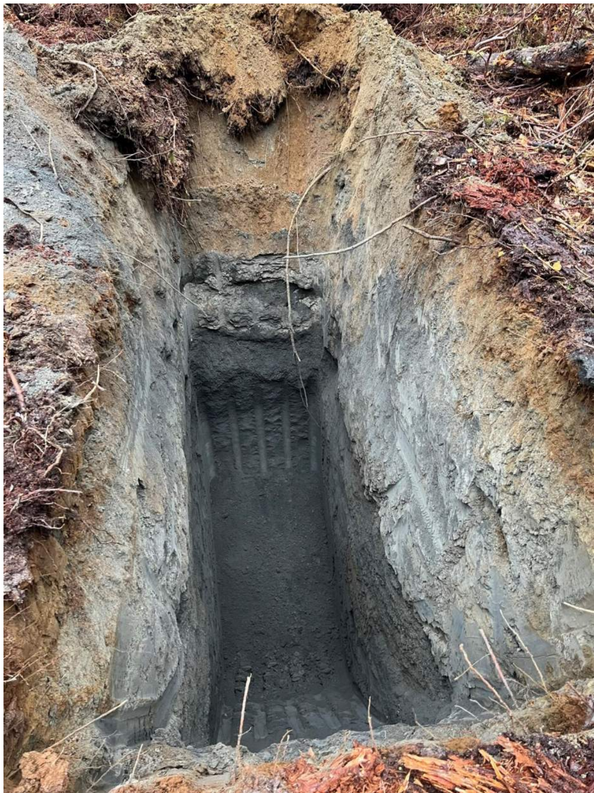
Photo A - 26: Test Pit TP26
