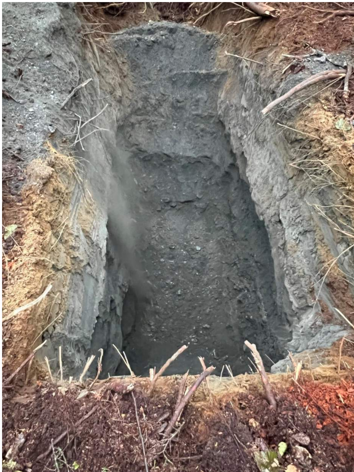
Photo A - 24: Test Pit TP24
