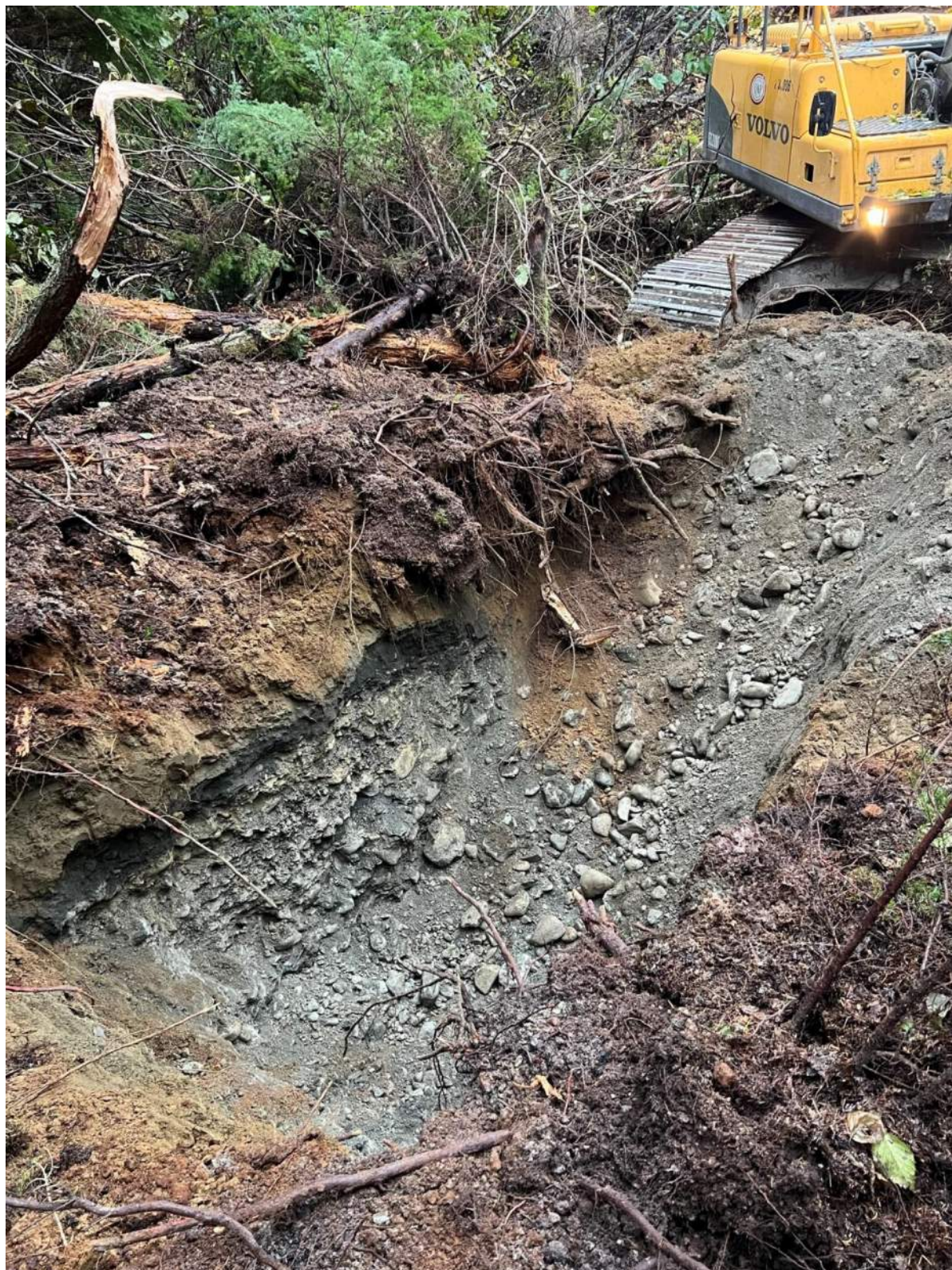
Photo A - 22: Test Pit TP22 In Progress
