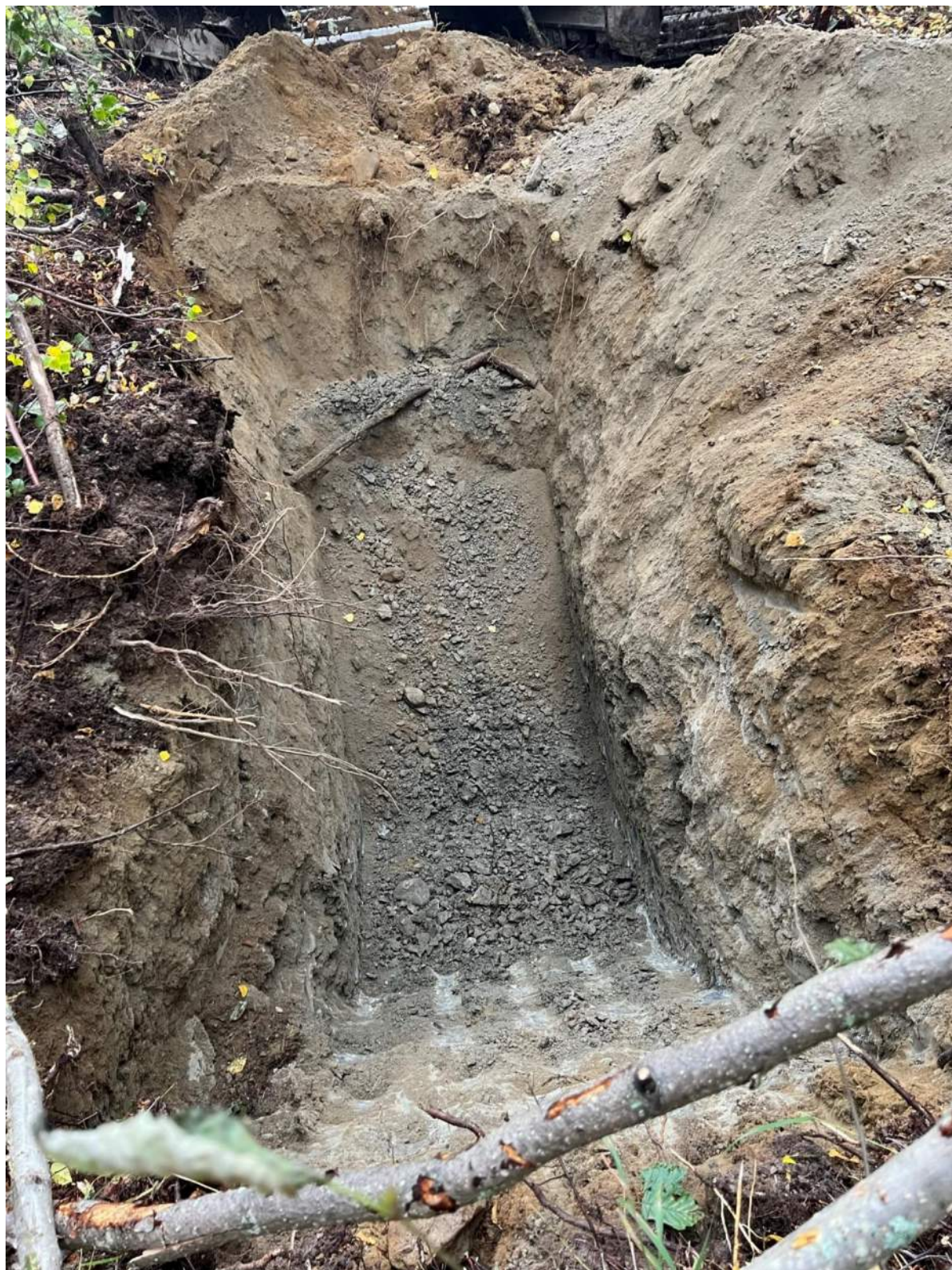
Photo A - 10: Test Pit TP10
