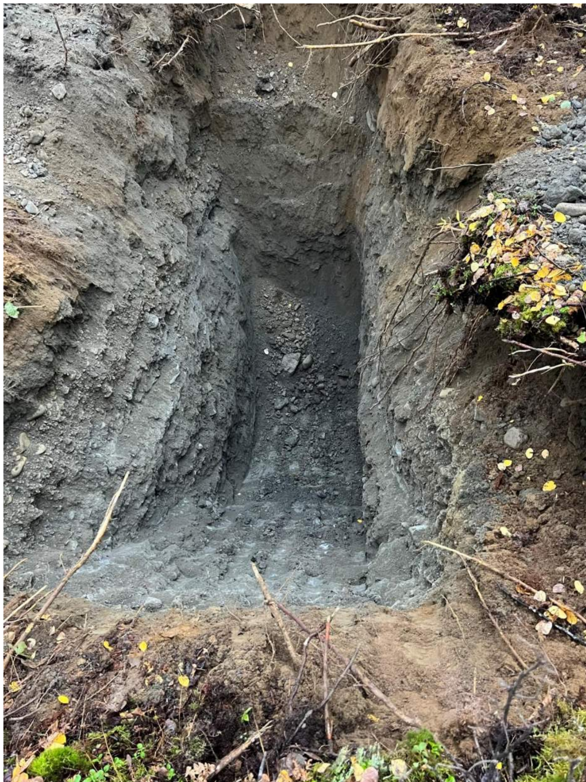
Photo A - 1: Test Pit TP1
