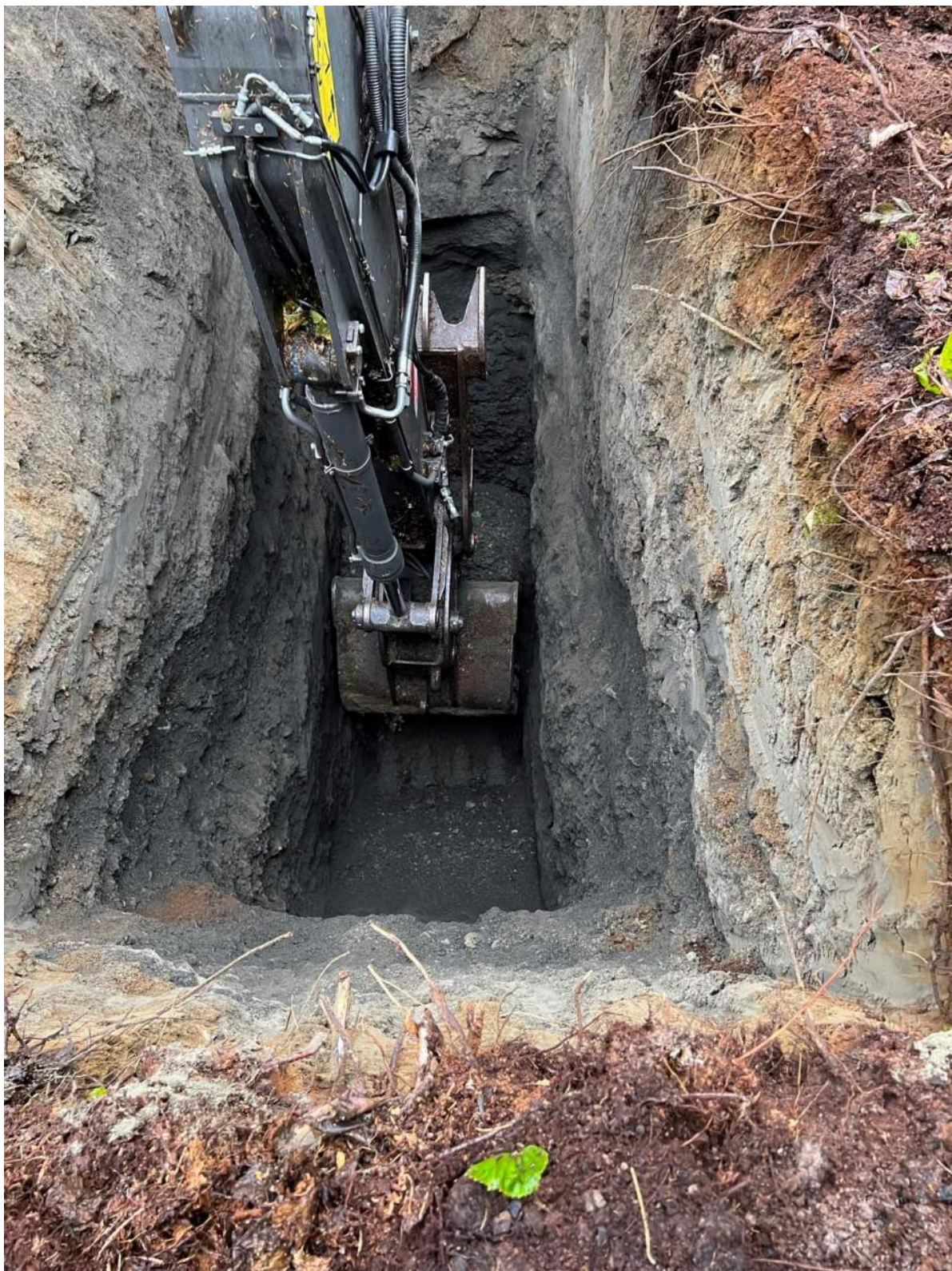
Photo A - 27: Test Pit TP27
