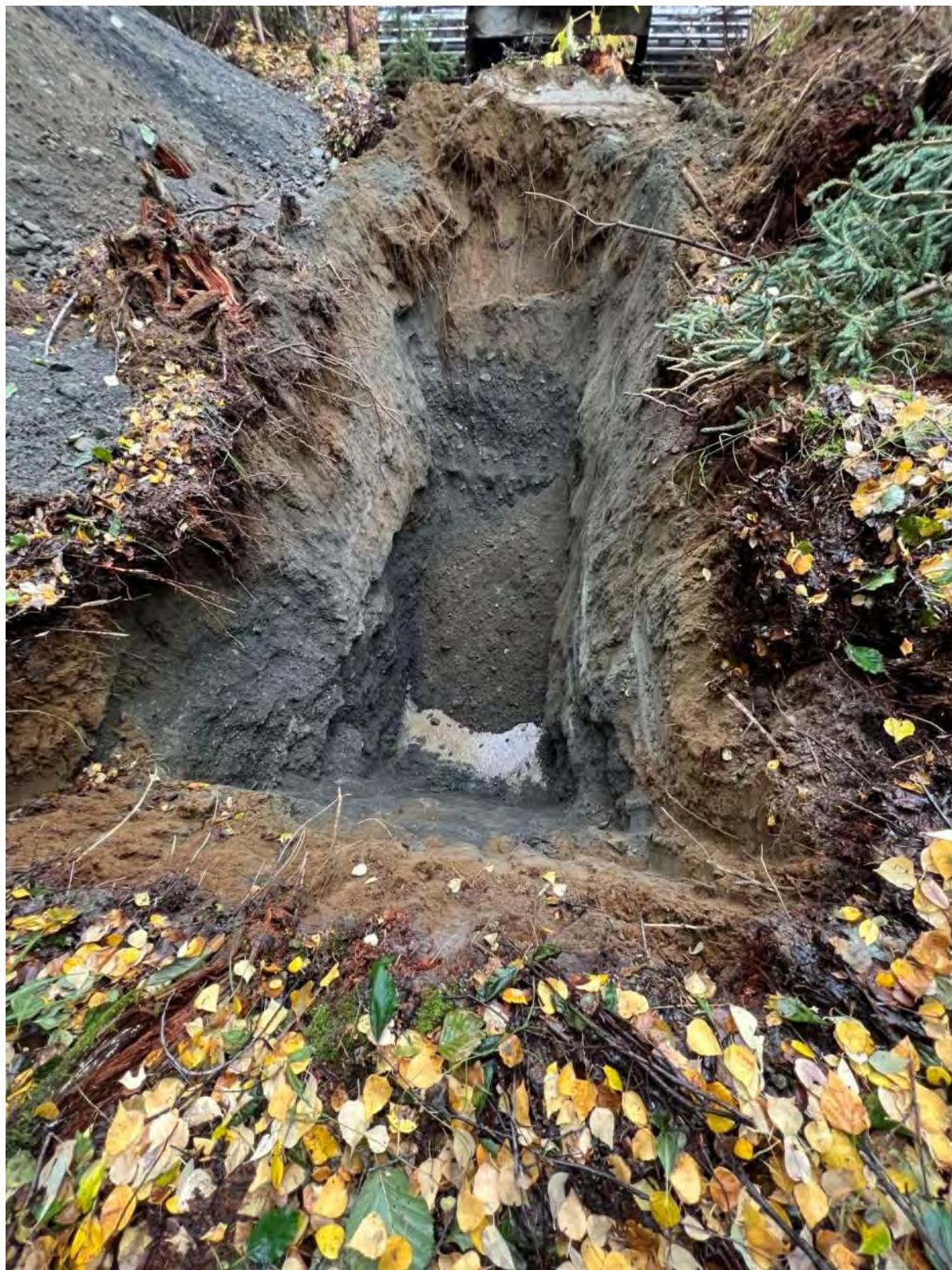
Photo A - 15: Test Pit TP15
