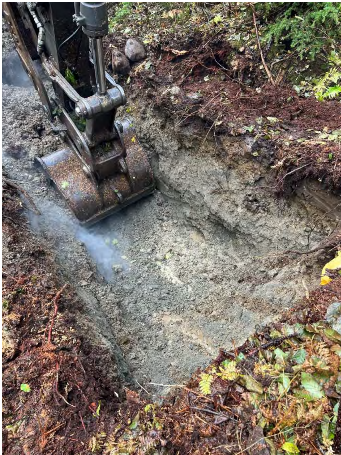
Photo A - 29: Test Pit TP29
