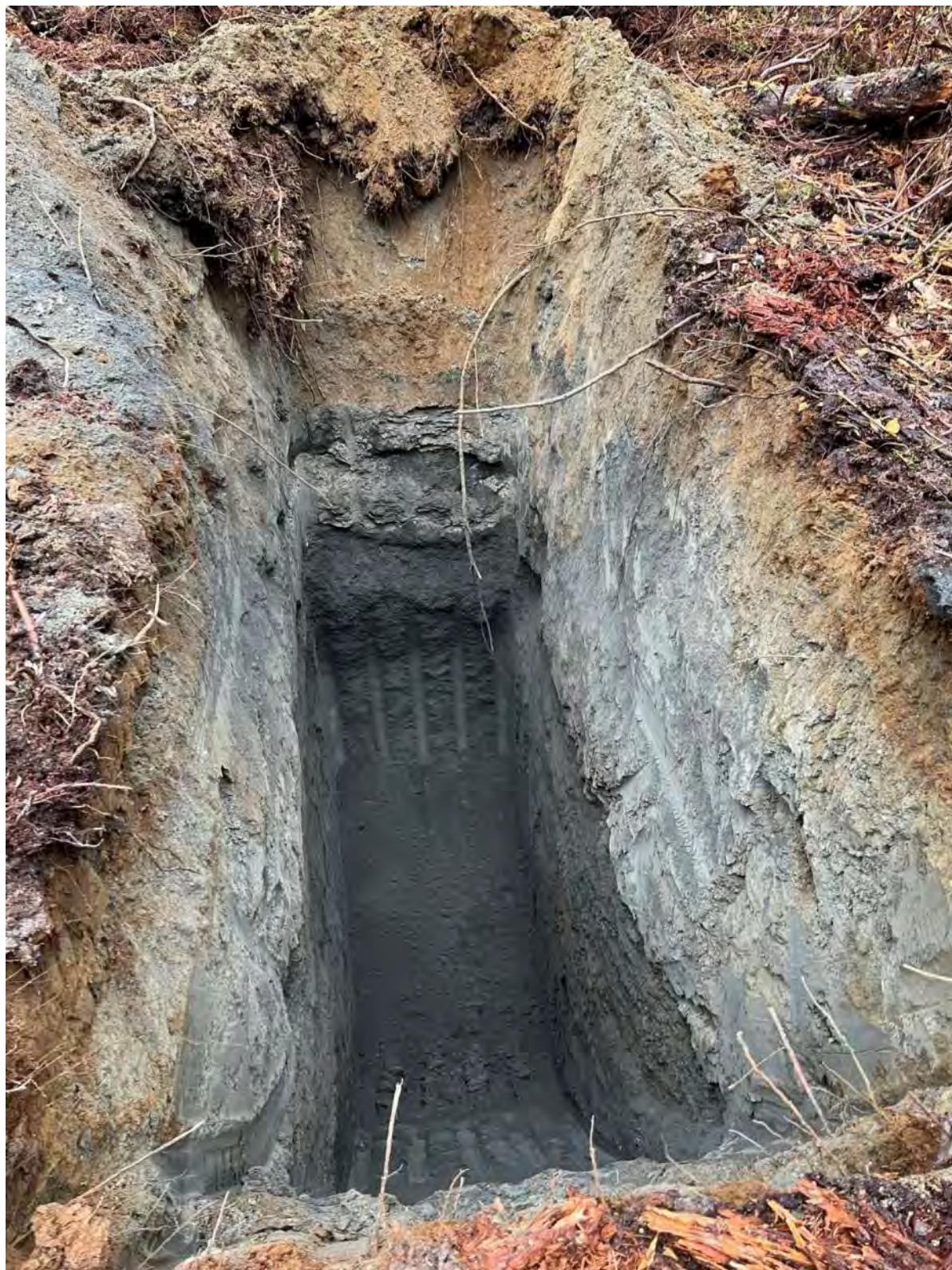
Photo A - 26: Test Pit TP26
