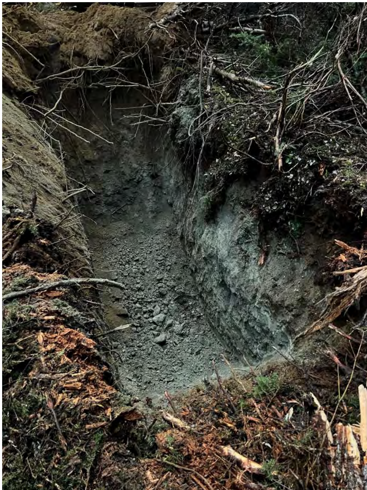
Photo A - 34: Test Pit TP34
