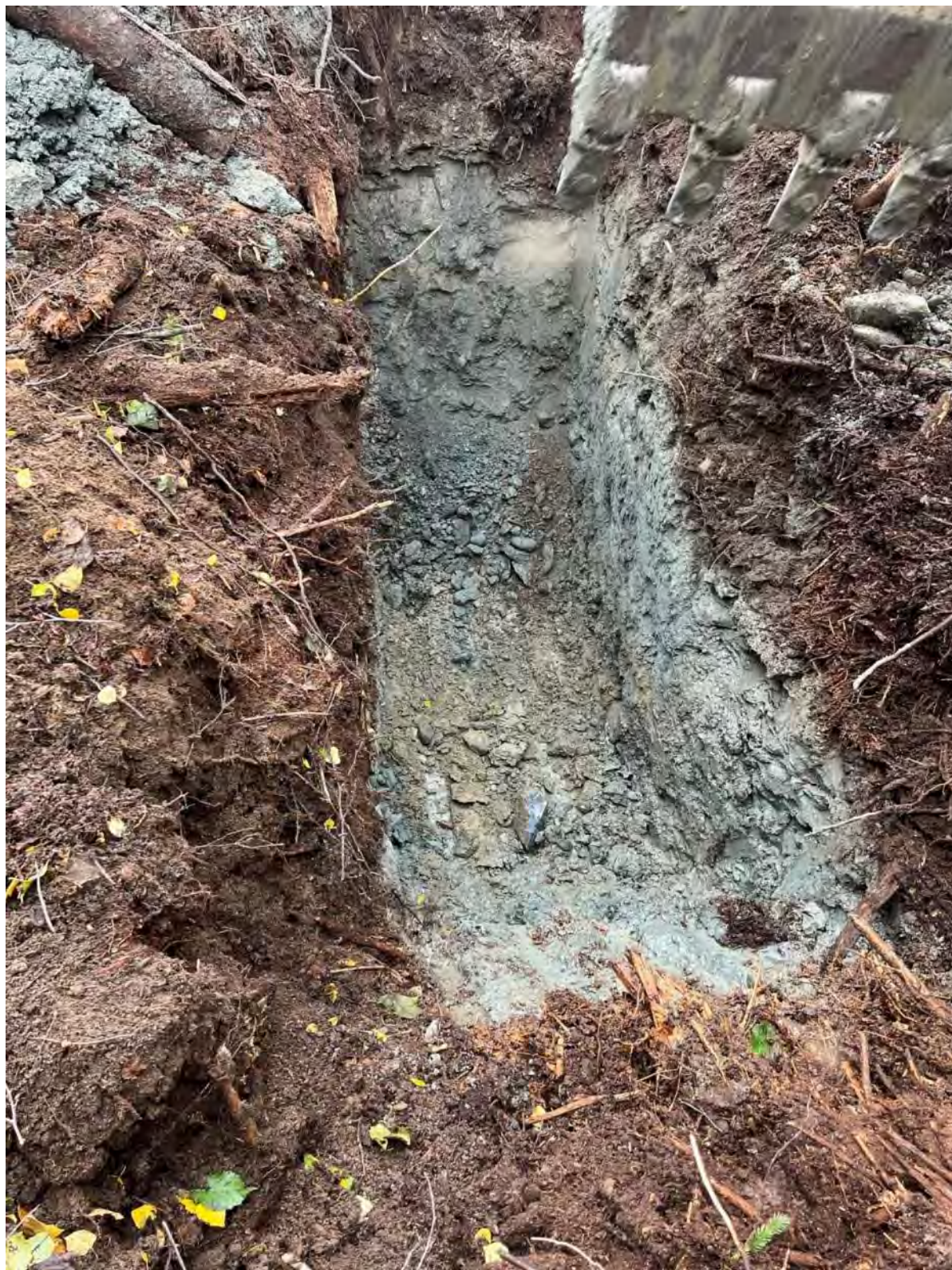
Photo A - 11: Test Pit TP11
