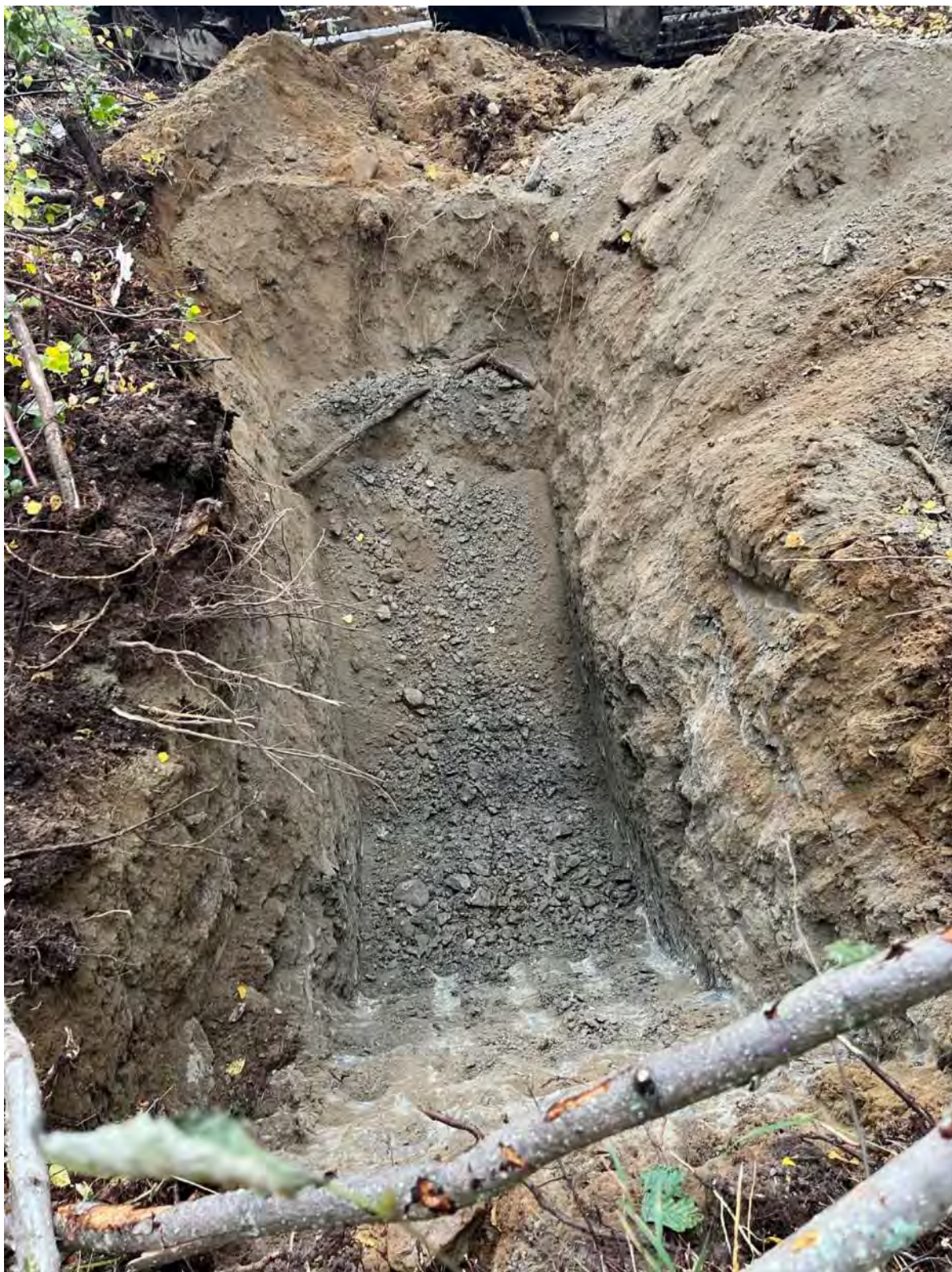
Photo A - 10: Test Pit TP10
