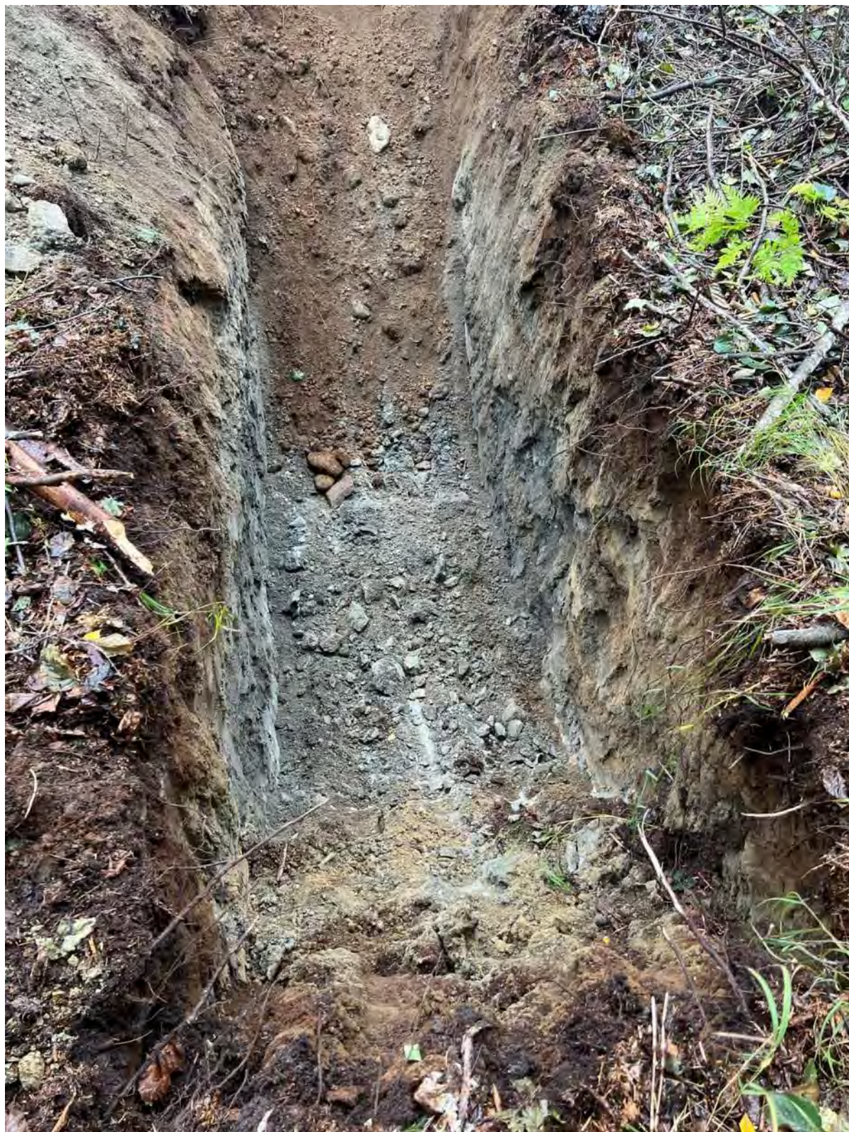
Photo A - 8: Test Pit TP8
