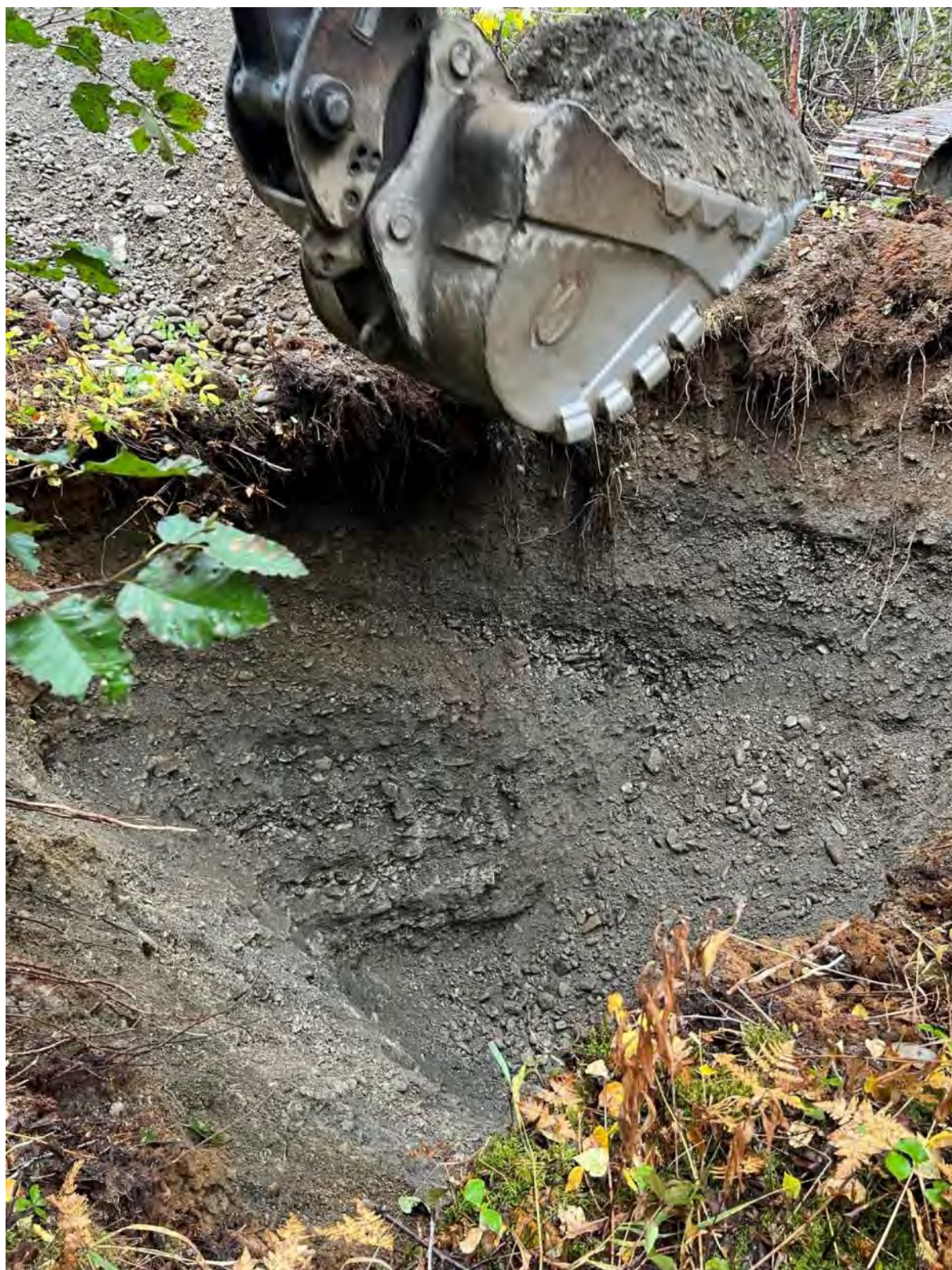
Photo A - 2: Test Pit TP2
