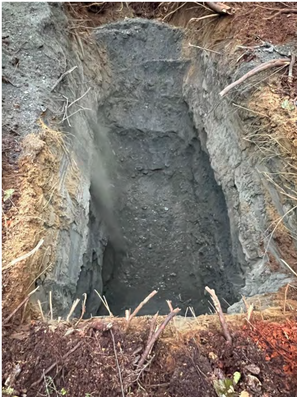
Photo A - 24: Test Pit TP24
