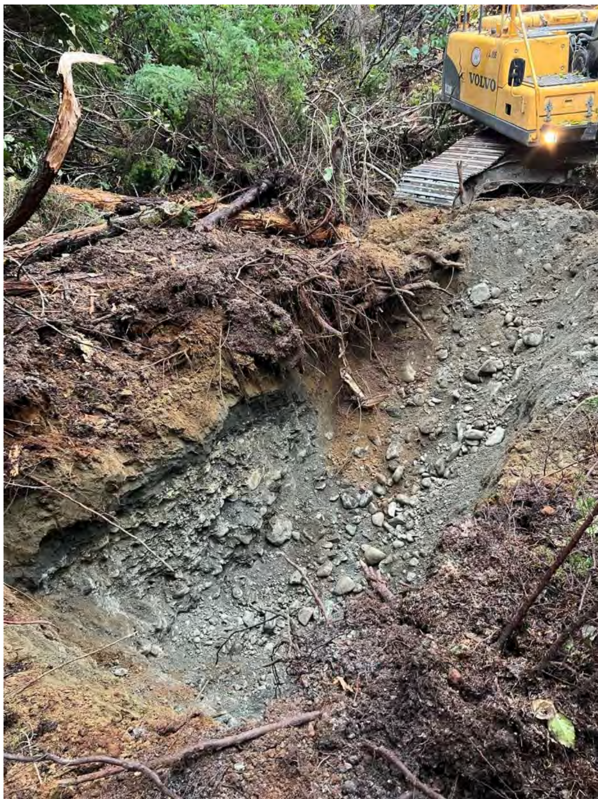
Photo A - 22: Test Pit TP22 In Progress
