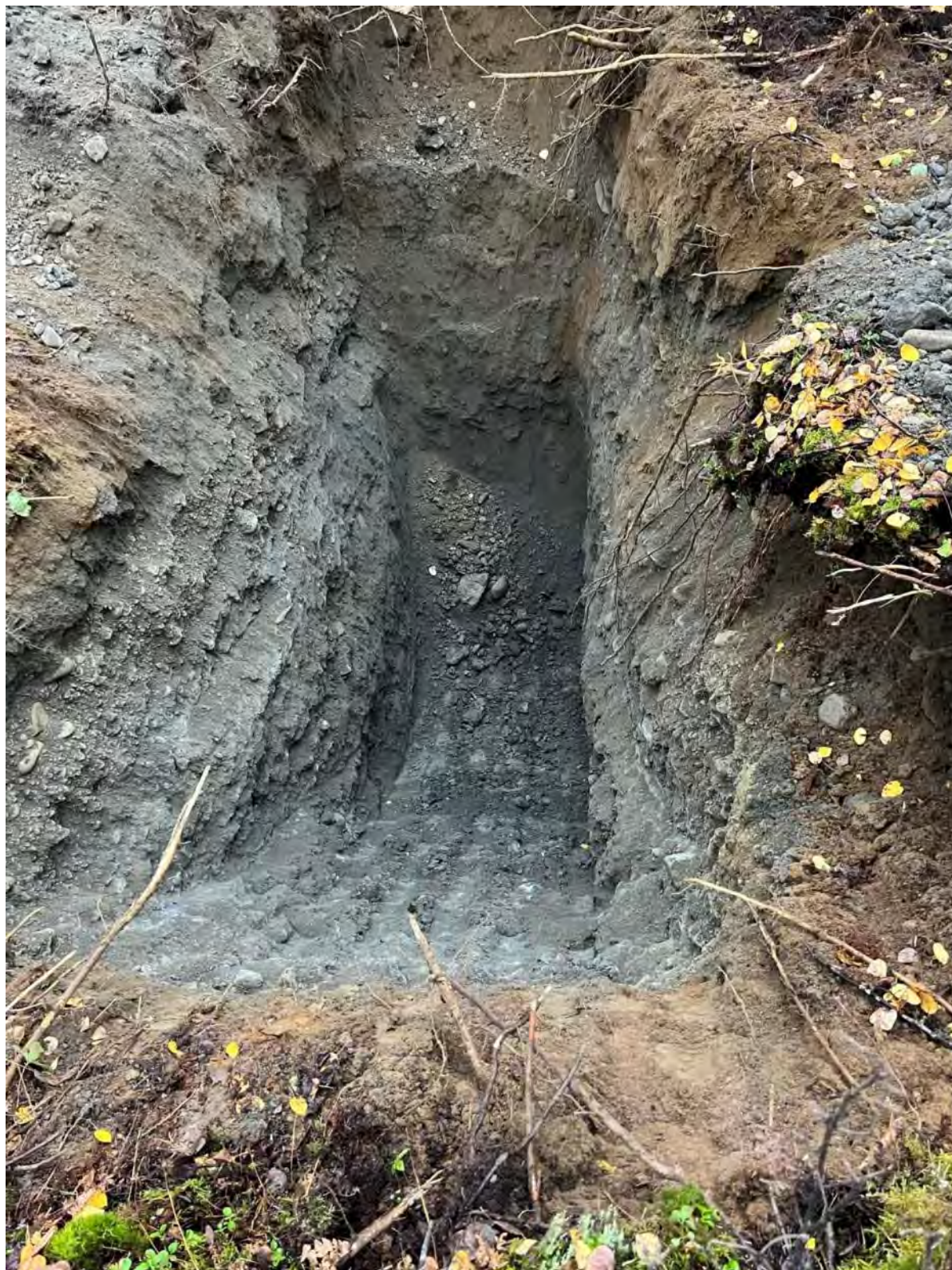
Photo A - 1: Test Pit TP1
