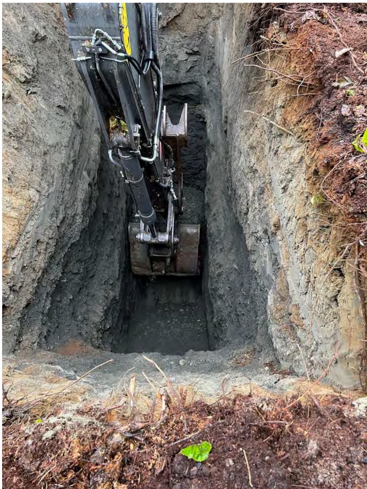
Photo A - 27: Test Pit TP27
