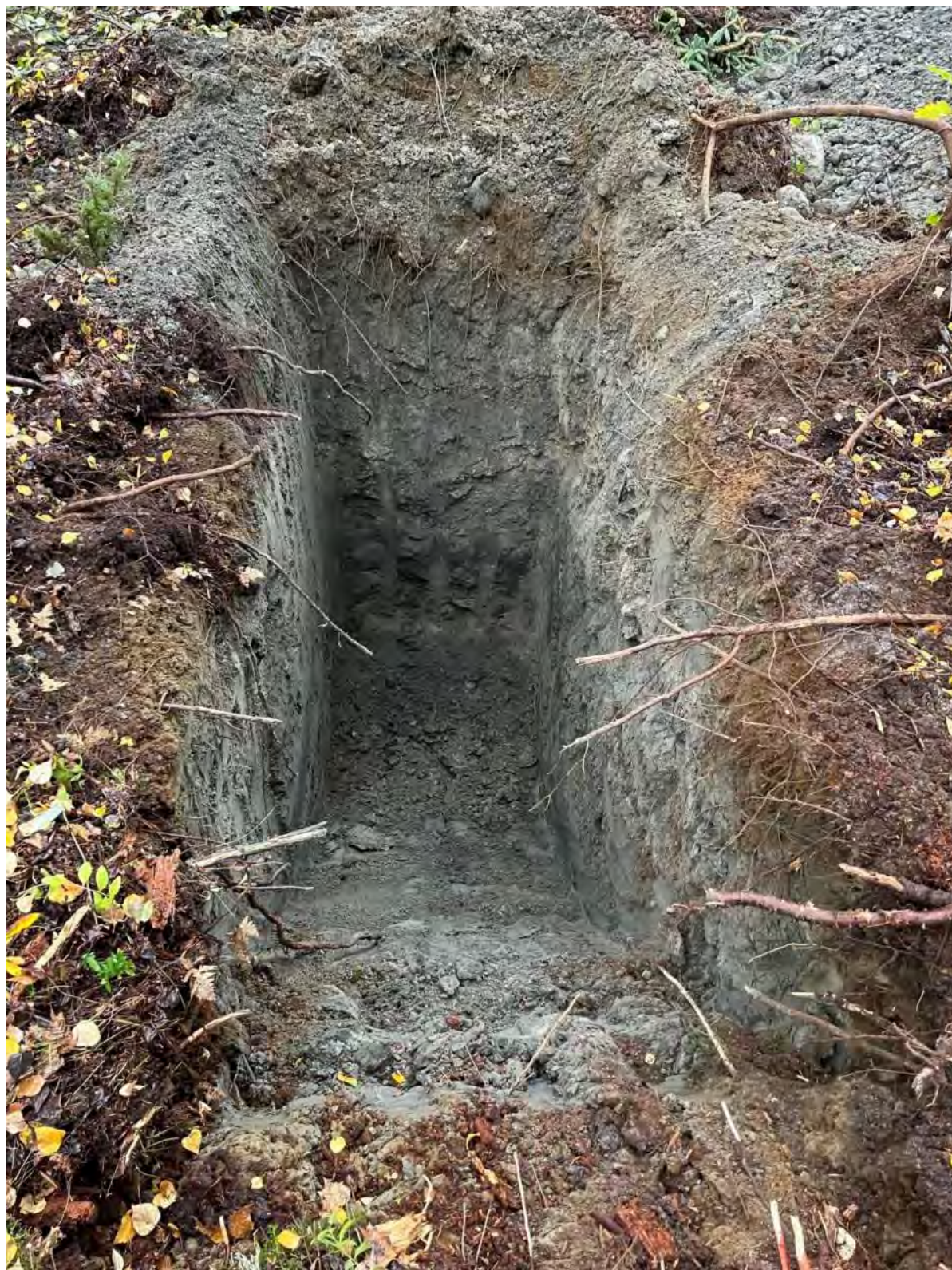
Photo A - 37: Test Pit TP37
