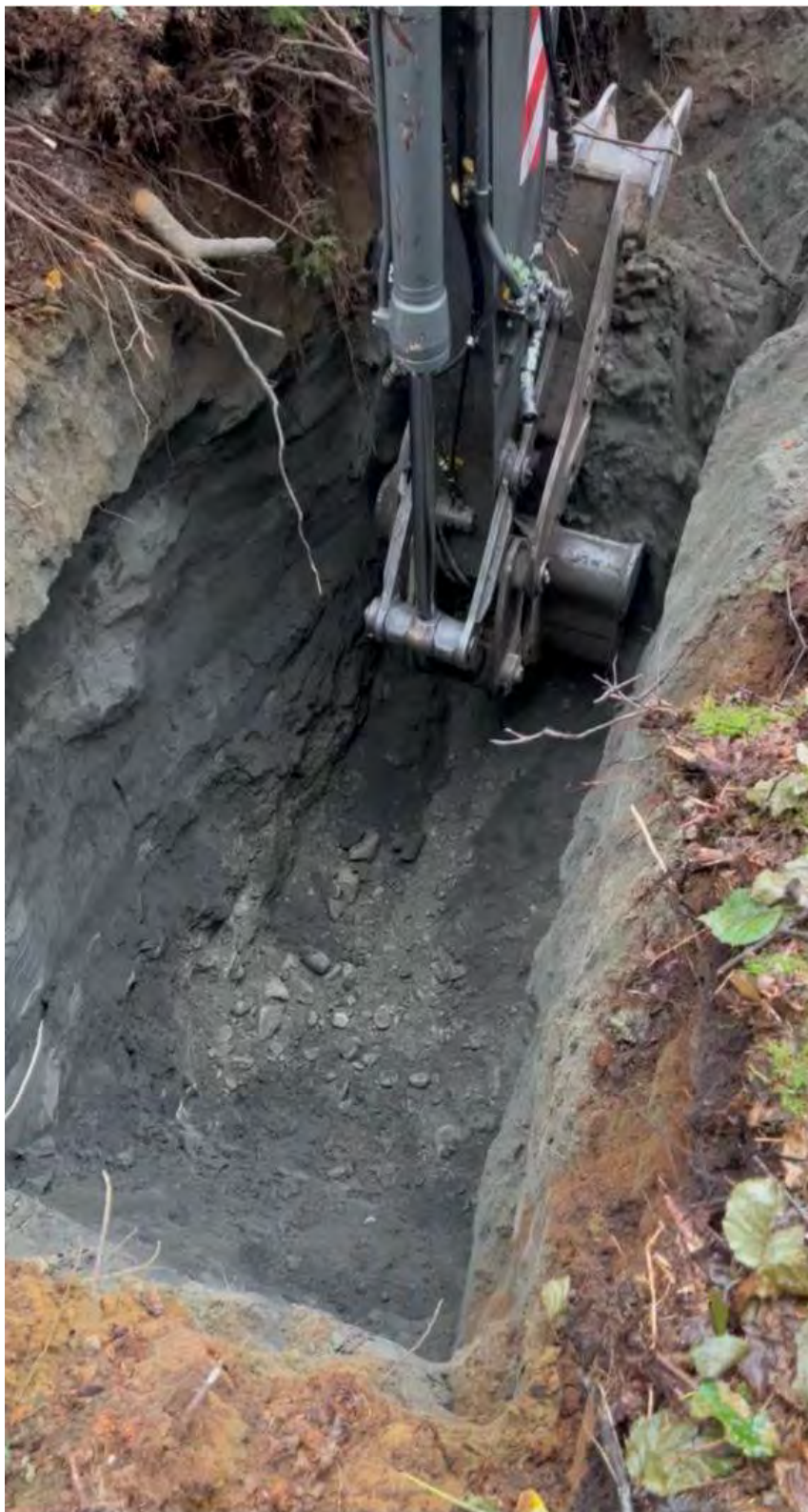
Photo A - 21: Test Pit TP21
