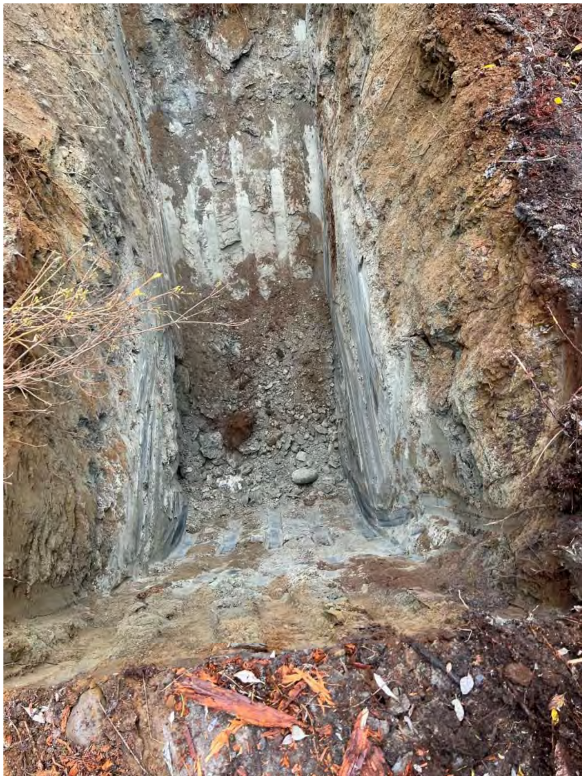
Photo A - 38: Test Pit TP38
