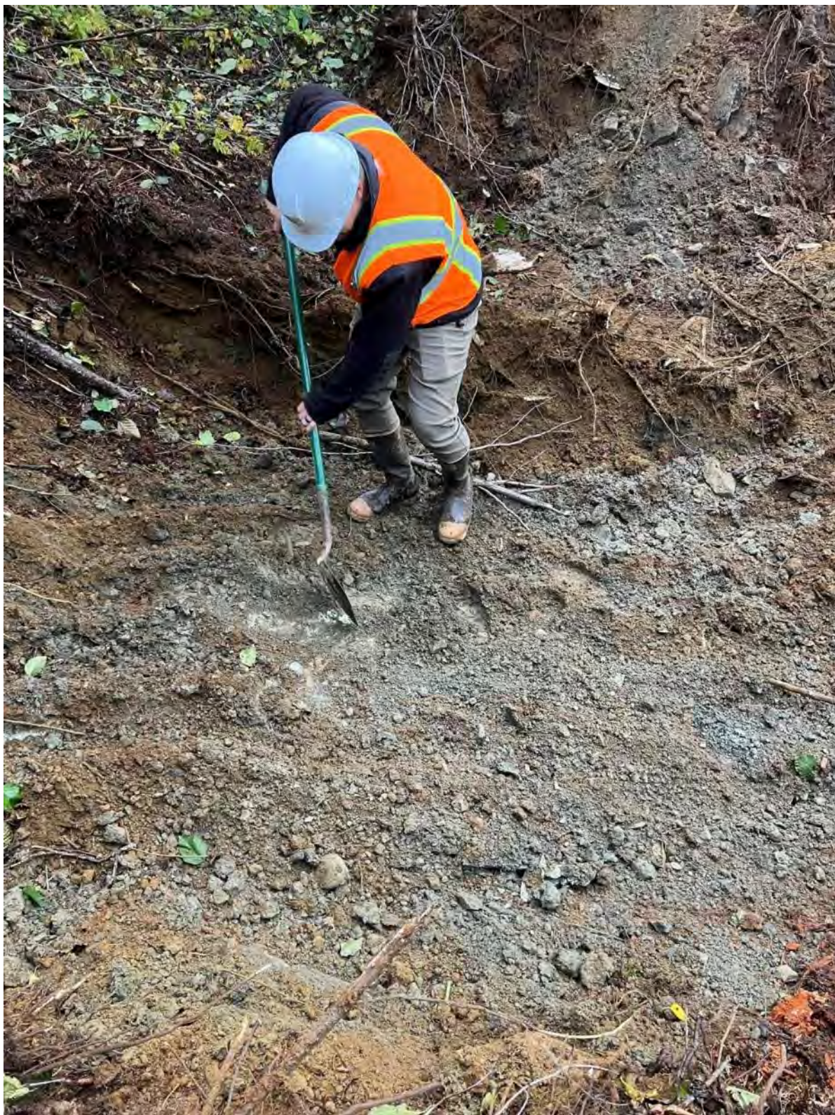
Photo A - 6: Test Pit TP6
