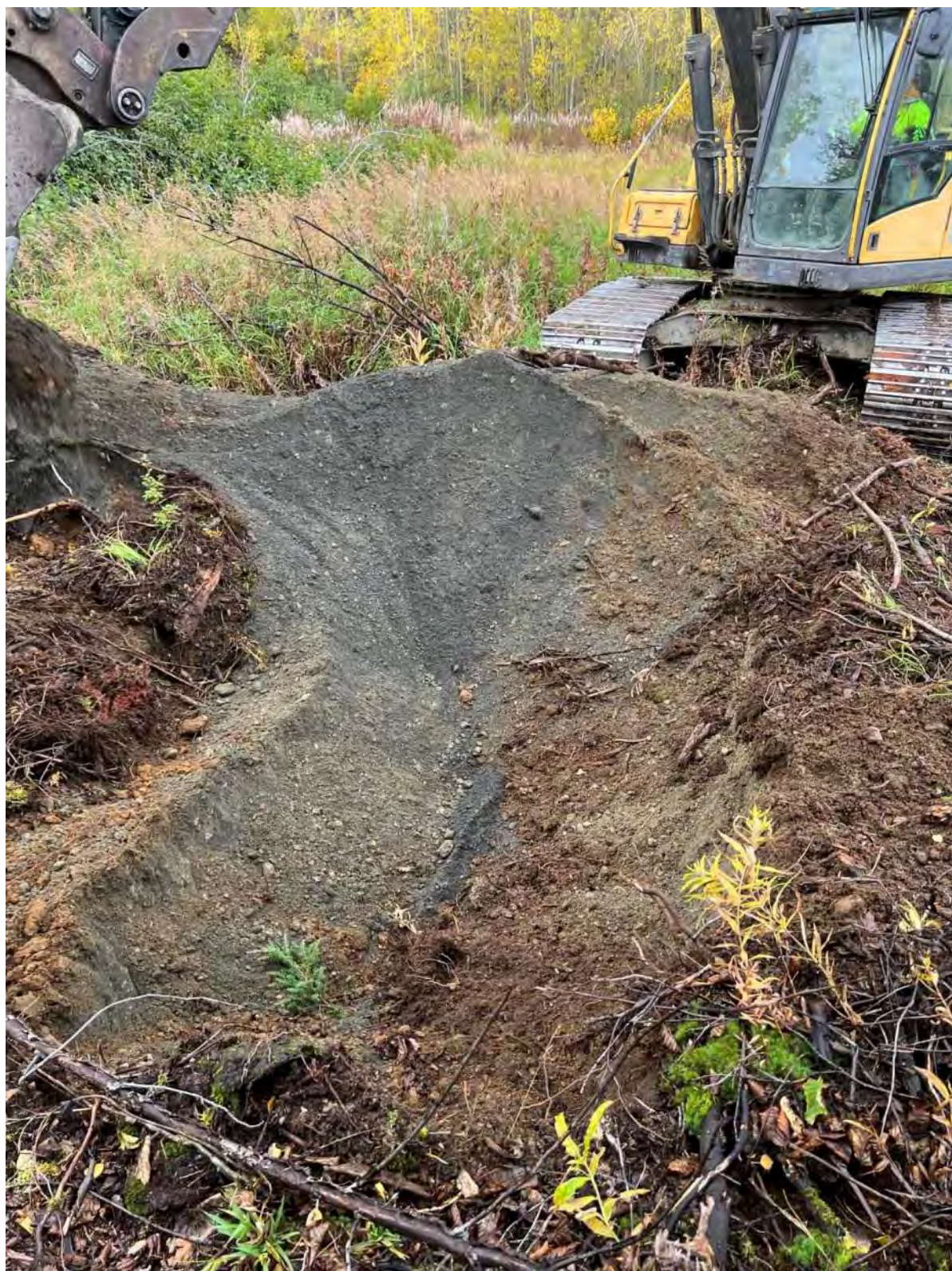
Photo A - 18: Test Pit TP18 In Progress
